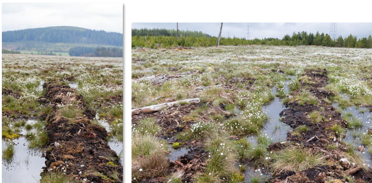
Figure 3. Example of backfill trenches at Gow moss. Note the positive indicators – the high water table and extent of cotton grass.
