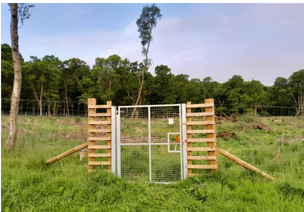
Example of self-closing pedestrian gate
