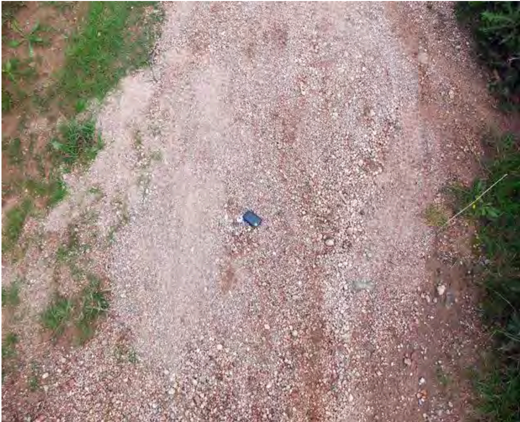
4. The key fob is to give an idea of the size of the fine gravel washed down the path.
