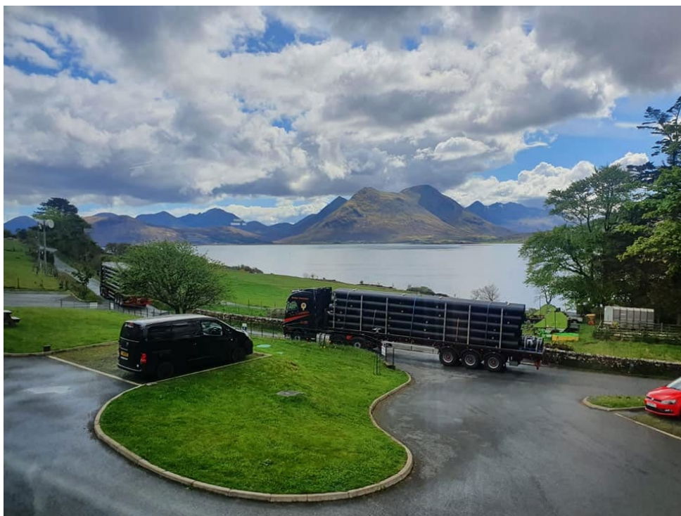
Pipework for Raasay Community Renewables hydro scheme arriving at Inverarish (Photo courtesy of Ross Gillies, Raasay Community Renewables)
