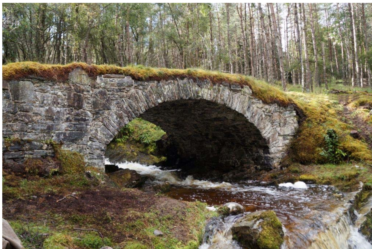
Bridge 009 (the NE bridge) after consolidation
